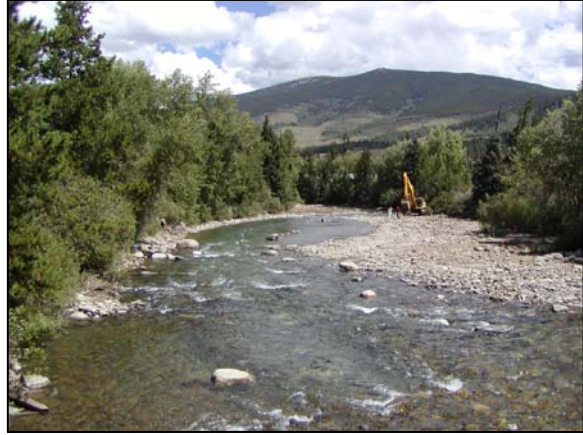
Photo 2 shows an enhanced section of the Blue River located at the Forest Service Building in the Town of Silverthorne. The channel section was reshaped creating a defined low flow thalweg (left) and exposed gravel bars (right). A riffle-pool-glide sequences along with instream habitat structure is evident in the center of the photo. ERC project 2005.
