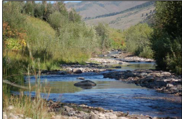
Photo 4 shows an enhanced section of a side-channel of the East River located at the Reserve (private fishing club) located in Crested Butte, Colorado. Constructed point bars and riffle-pool-glide features are seen in the photo. ERC project 2006.
